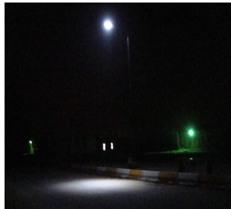
FIGURE (17) PHOTOGRAPH OF THE HIGH POWER LED LAMP WITHOUT LENS MOUNTED IN THE FIXTURE ON THE POLE DURING THE NIGHT
