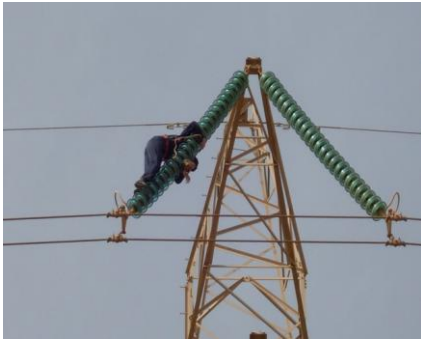
Figure (7): hand washing of 220 kV line insulators
