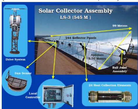
Fig (1.4): The main components of Parabolic Trough system (Source: H. Price, 2006)
