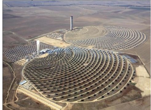
Fig. 2 Central receiver (Power Tower)
